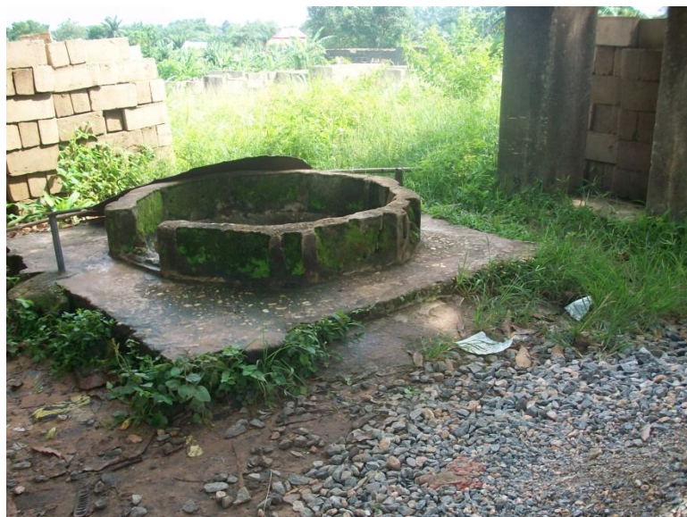
Fig. 2: Typical monitored well at Ugep
