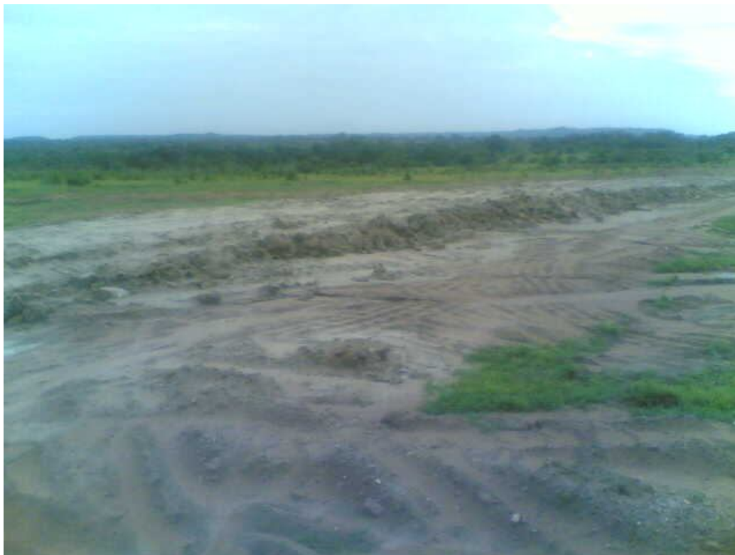
Fig. 4: Construction activity for expansion of irrigation scheme
