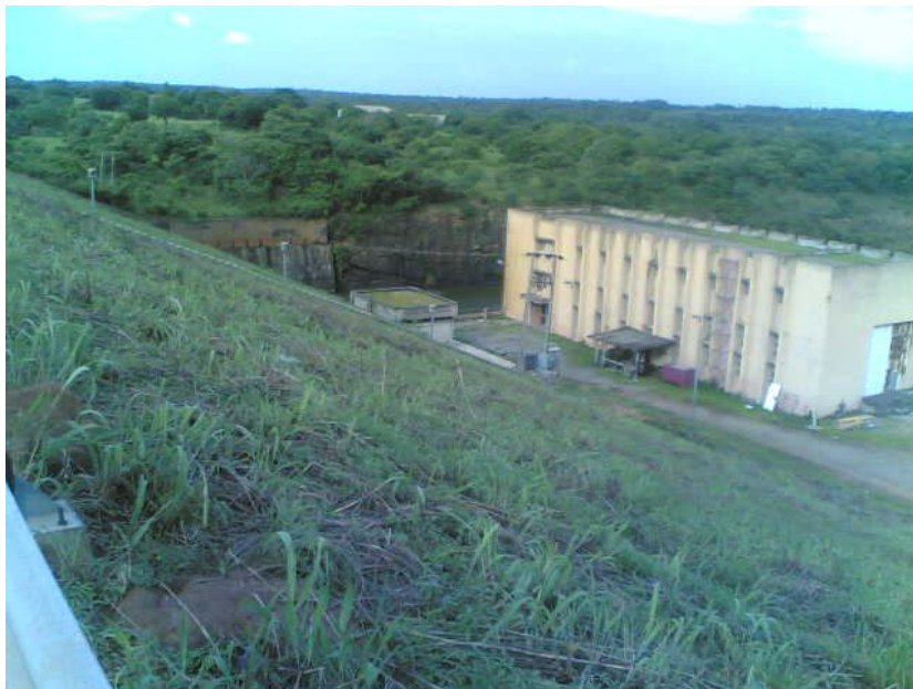
Fig 2: Oyan Dam Downstream Face showing Hydropower Building
