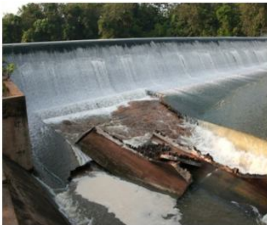
Fig. 5: The UI Dam Embankment and Spillway after the flood 6 th September 2011
