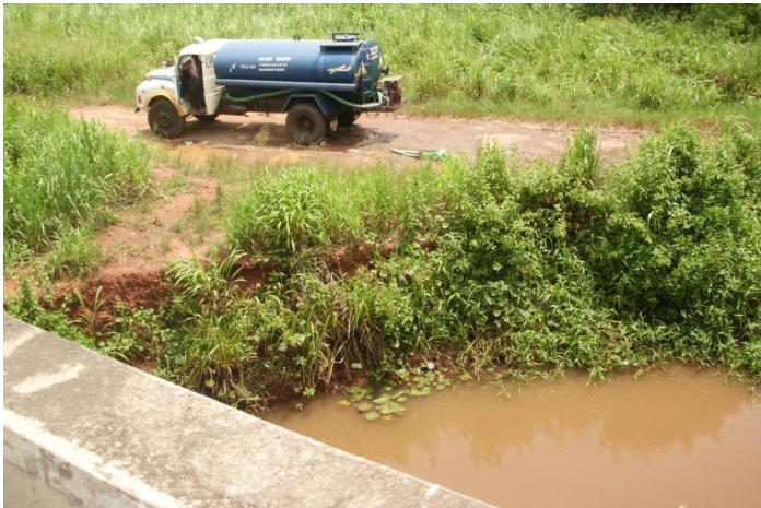
Figure 8: River Owiwi at the bridge on Abeokuta – Lagos road
