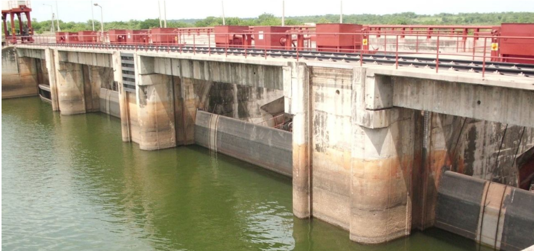
Figure 3: Spillway section at Oyan dam.
