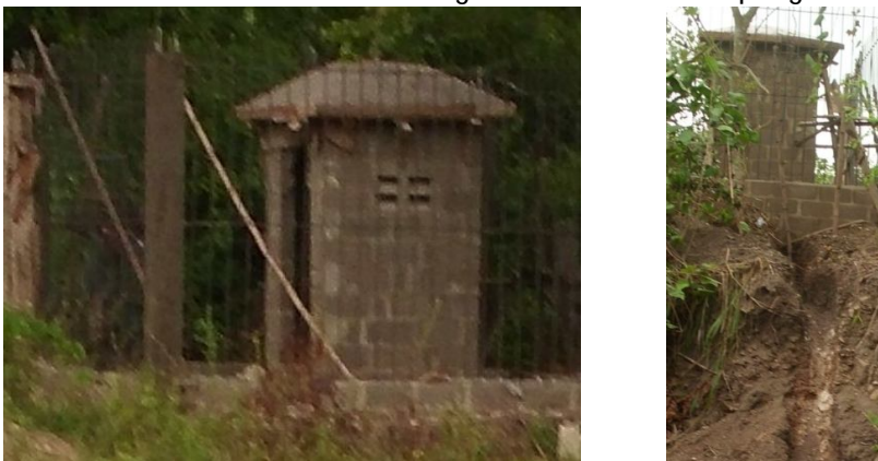
Figure 4: Early Flood warning equipment housing under construction
