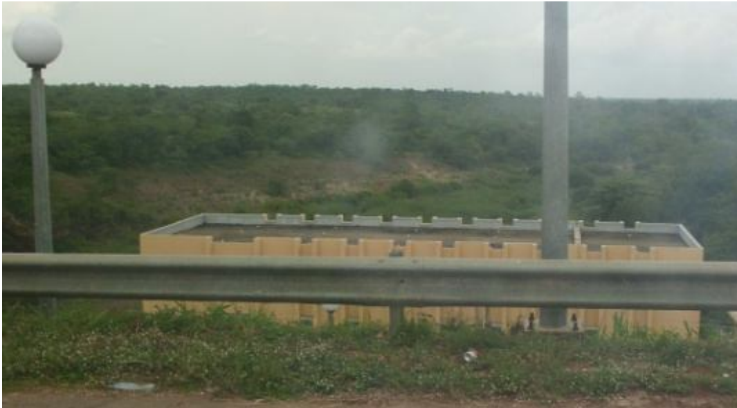
Figure 2: Power station at Oyan dam
