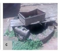
Figure 2: Construction patterns of selected wells - a: protected well; b: semi-protected; c: unprotected well
